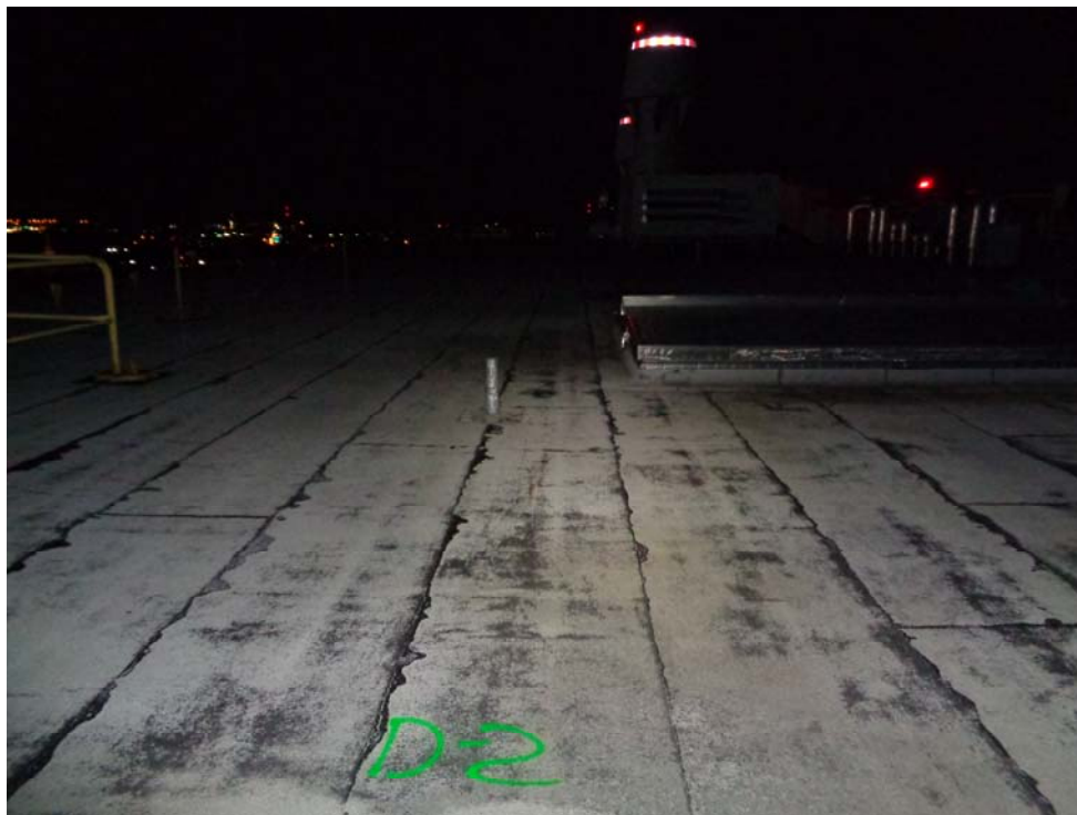
Roof D-Suspected wet area D-2, Southeast corner, looking West
