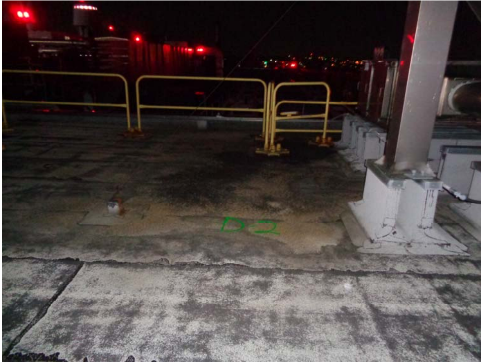
Roof D-Northeast corner, suspected wet area D-2, looking West
