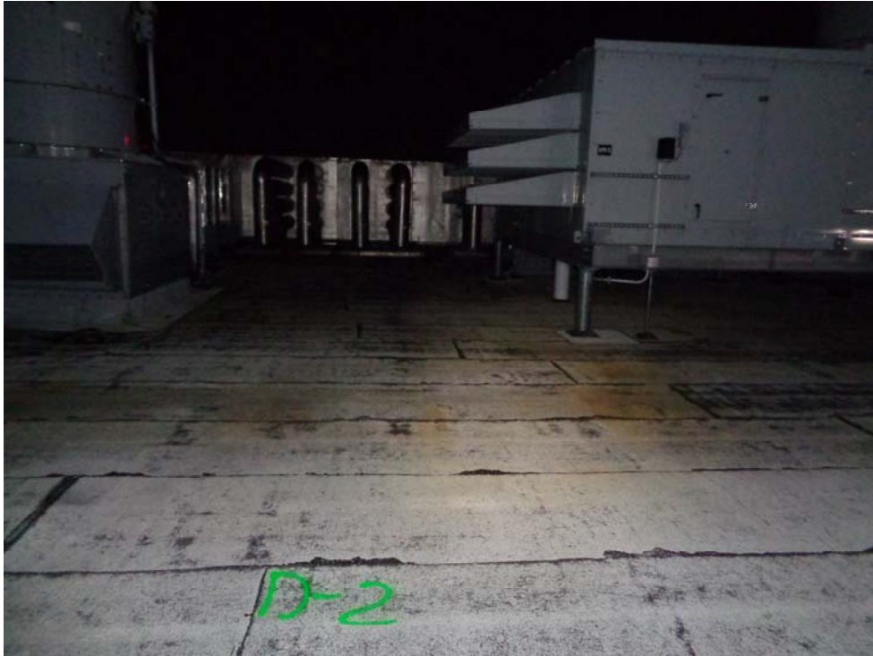
Roof D-Suspected wet area D-2, West side center, looking North
