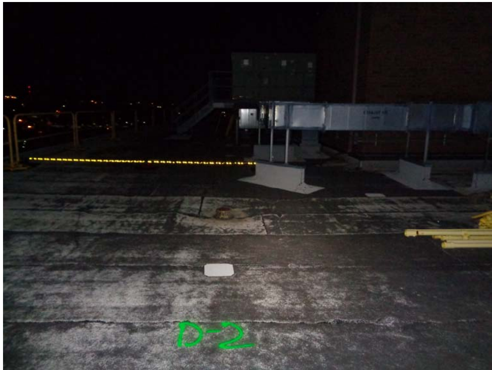
Roof D-Suspected wet area D-2, Southwest corner, looking North
