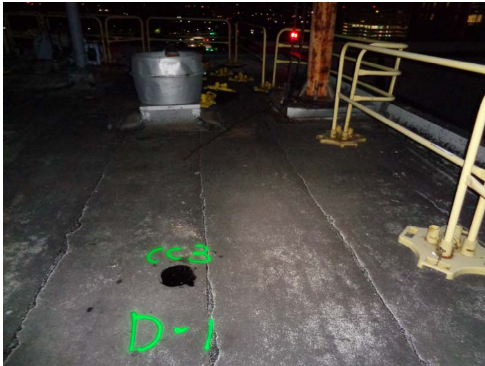
Roof D-Core cut #CC3 repaired, looking North
